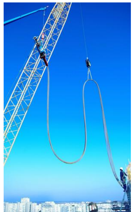
▲ Installation of a SLU-330 strand jack at the pressure ring
