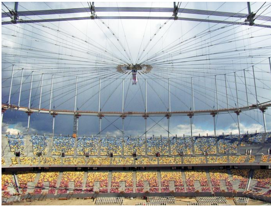
▲ The cable net structure in its final position
