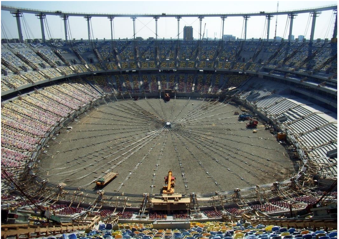
▲ The cable net structure was laid out before the lifting operation.
