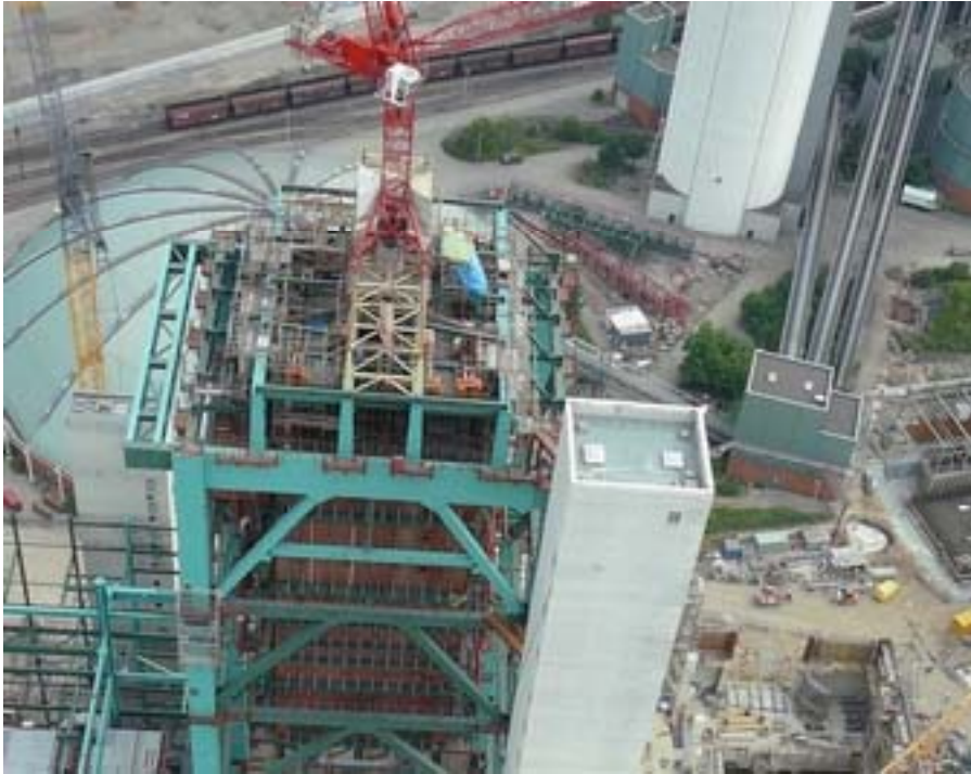
▲ Building the boiler house involved extensive use of strand lifting equipment.
