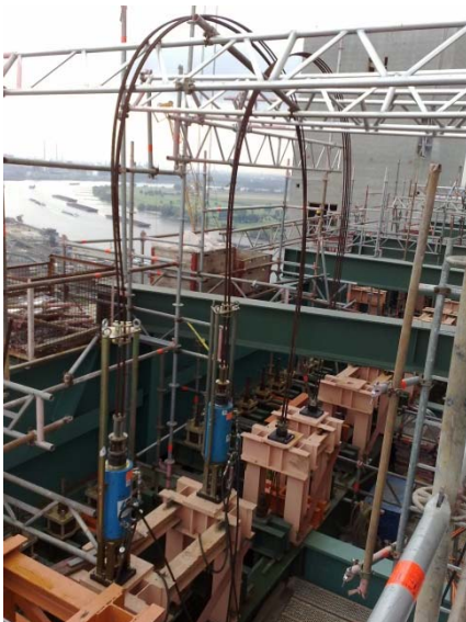
▲ Strand lifting units were installed to position over 6,000t of components.
