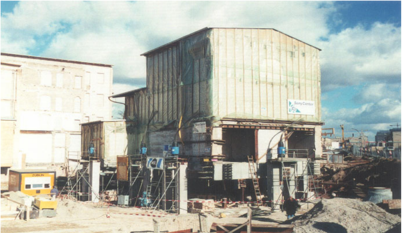
▲ Kaisersaal building on concrete frame, during the lifting
