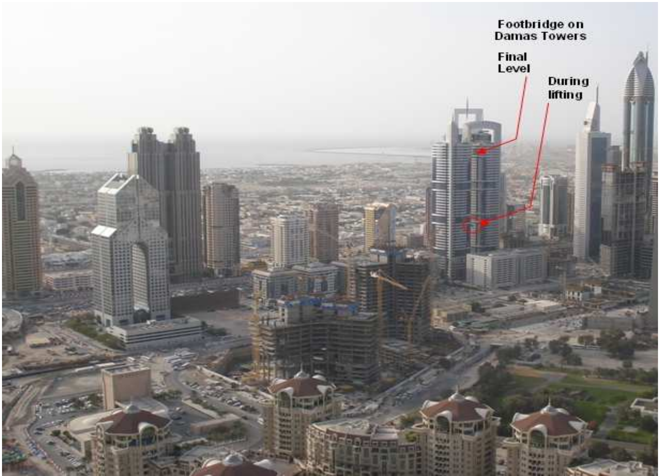
▲ Footbridge during lifting to final height of 165m
