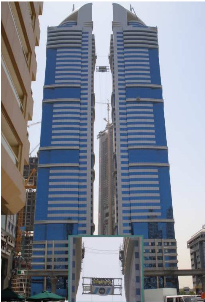
▲ Oversight and detail of Damas Tower Footbridge
