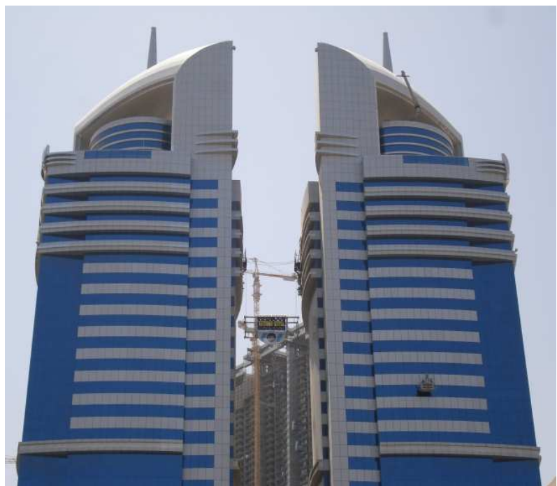
▲ Footbridge reaching final position
