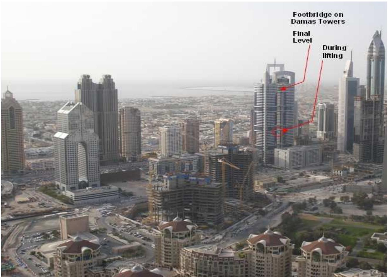
▲ Footbridge during lifting to final height of 165m
