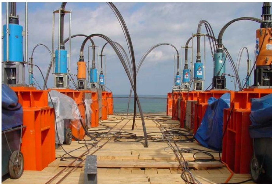
▼ Arrangement of VSL lifting units for boiler installation
