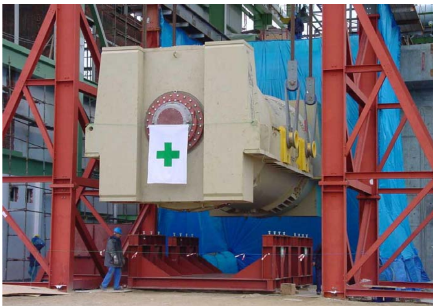
▼ Arrangement of VSL lifting units for boiler installation
