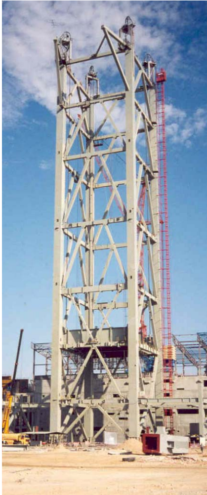
▲ The boiler frame during lifting of the suspension grillage
