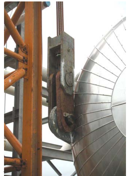
▲ Detail of lifting lug of deethanizer tower
