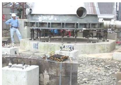
▲ Deethanizer tower lowered onto foundation
