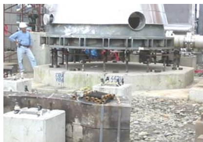
▲ Deethanizer tower lowered onto foundation
