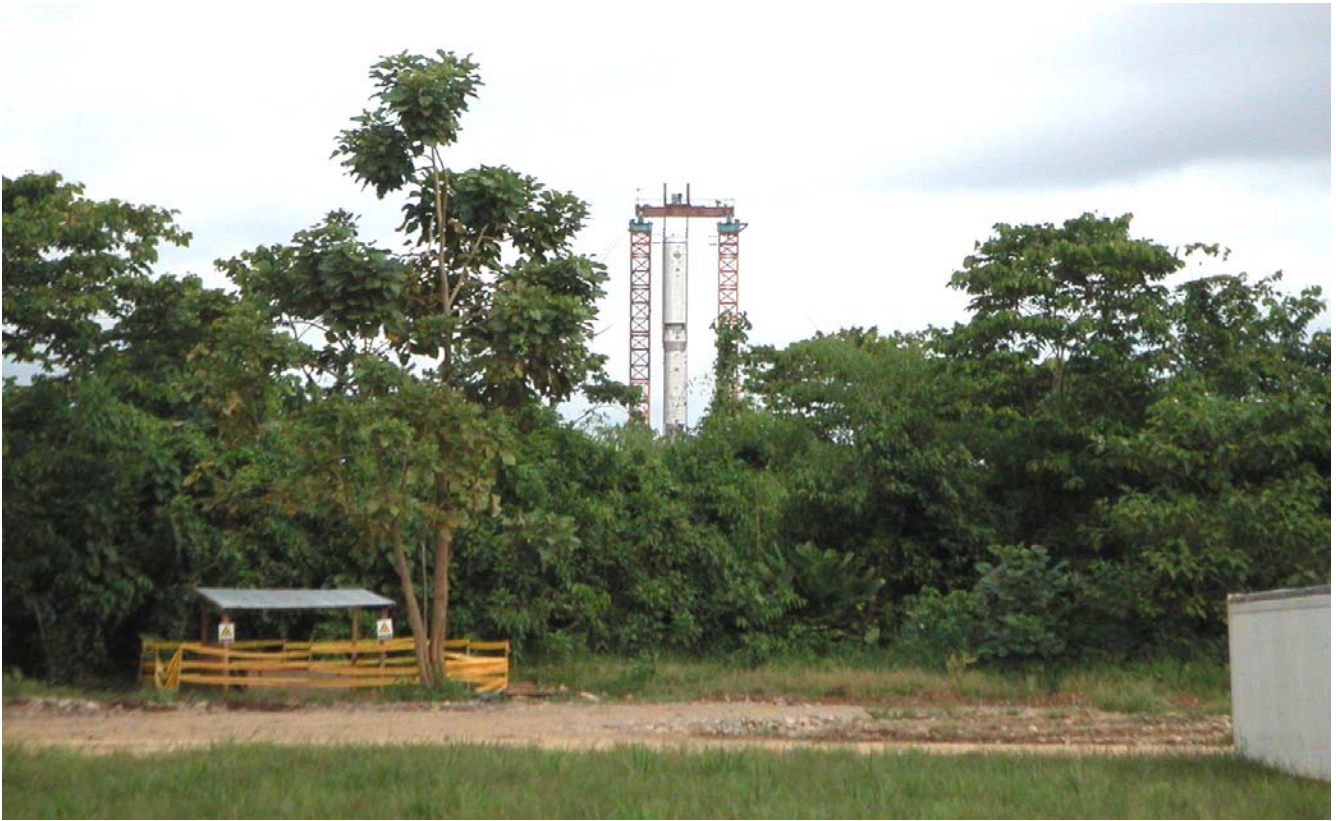
▲ Front view of the heavy lifting
