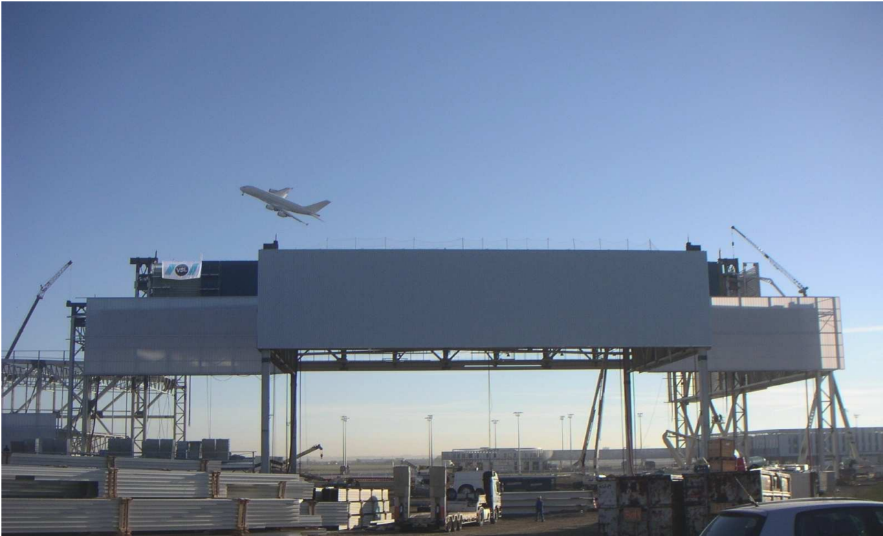
▲ Building site in Toulouse – France, erection of hangar
