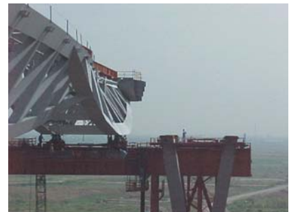
▼ Super Truss during slide
