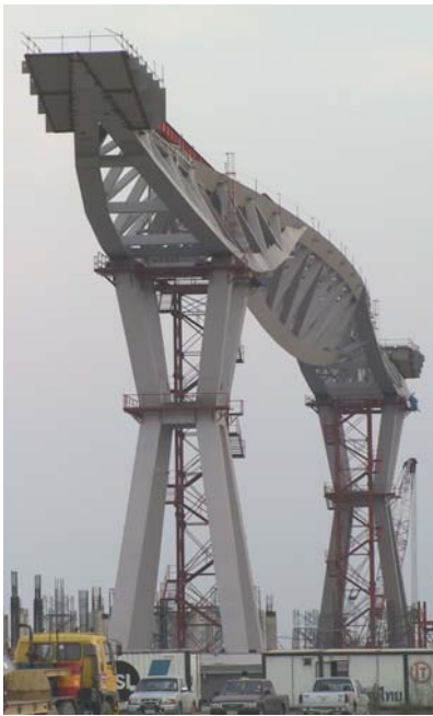
▲ Completed frame of supertruss and pylons
