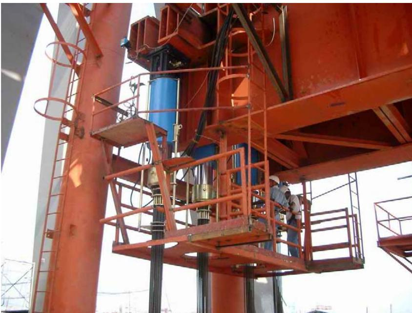
During the whole operation the Super Truss rested on sledges. These were equipped with hydraulics to allow movement and rotation in all directions. The advanced features of the lifting installation allowed for positive load distribution control and a final adjustment of the Super Trusses within millimetres.
