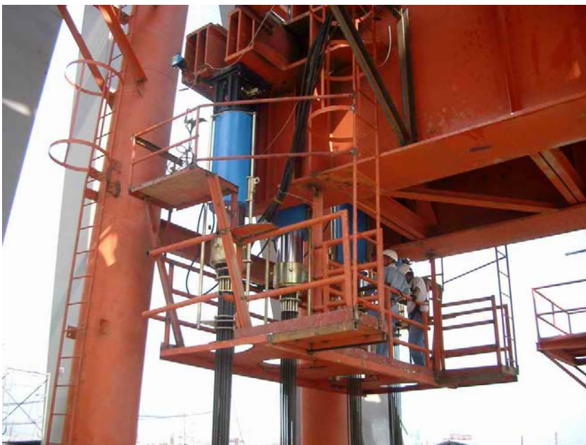
▼ Inverted Strand Lifting Units attached to the support beam, climbing up the static lifting cable
