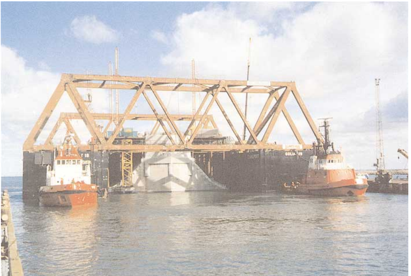
▲ Caisson hanging on lifting strands between two barges being towed out of fabrication dock.
