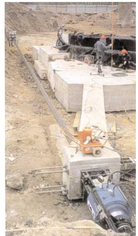
▲ The ski-shaped metal sheets acted as launching pads
