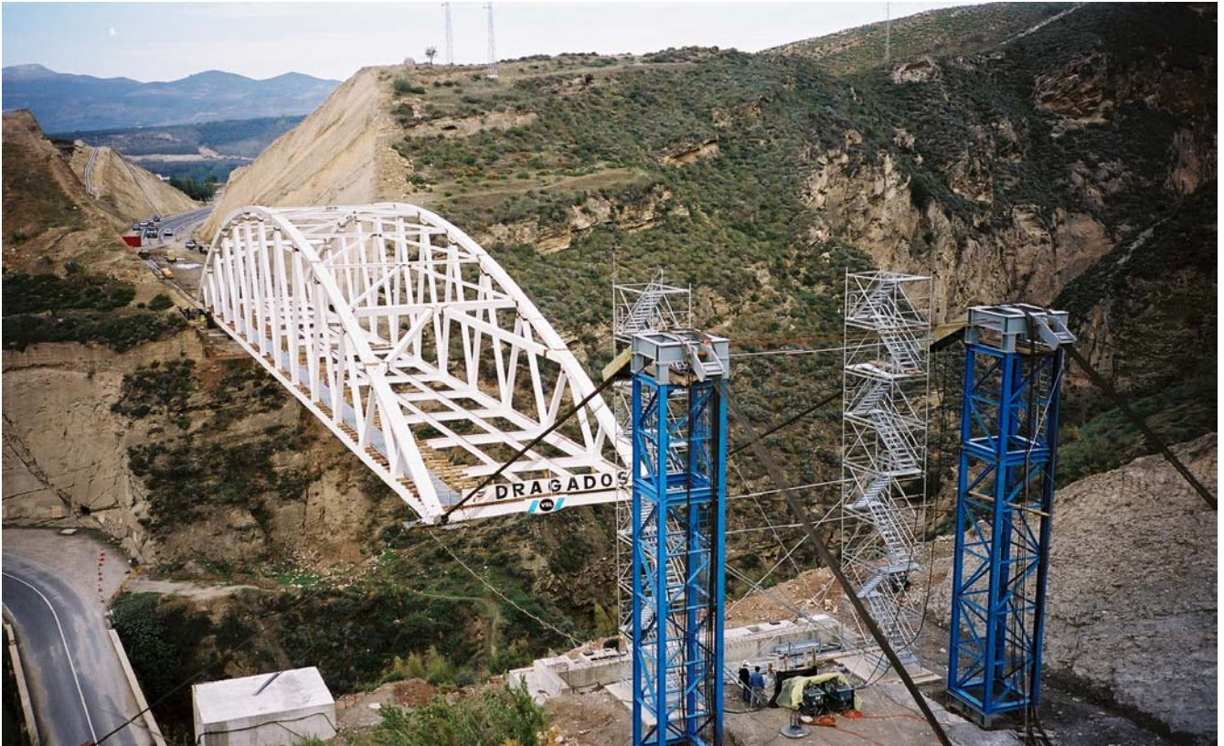
▲ General view of the structure
