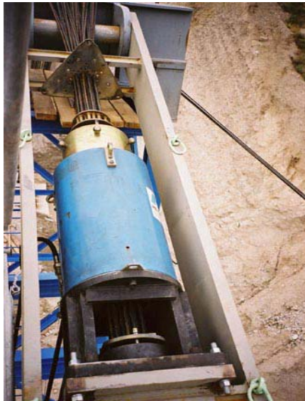
▲ Main cable unit type VSL SLU 440 on a hinged frame
