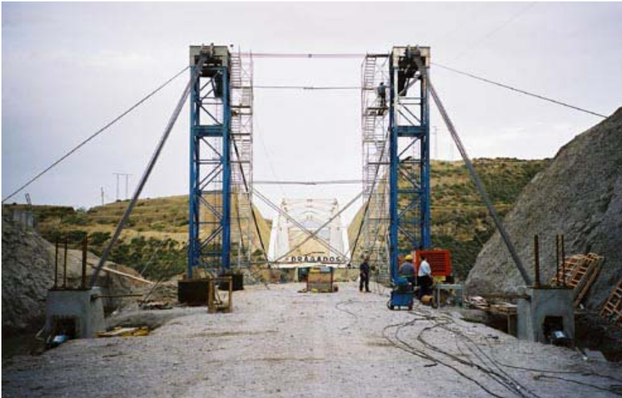
▲ Main cable unit type VSL SLU 440 on a hinged frame
