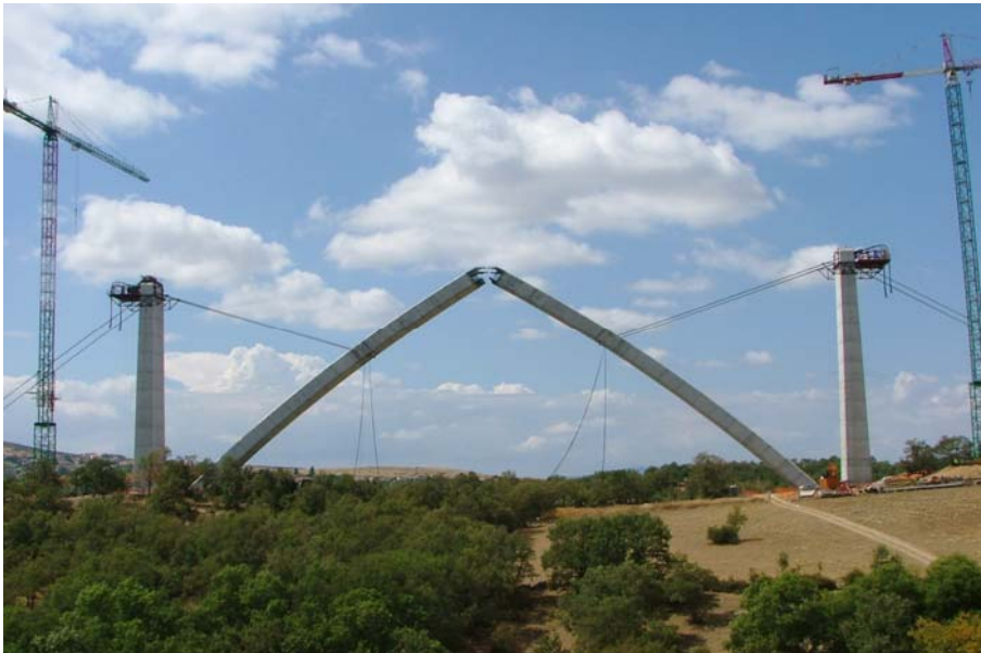
▼ Half arch initial construction position
