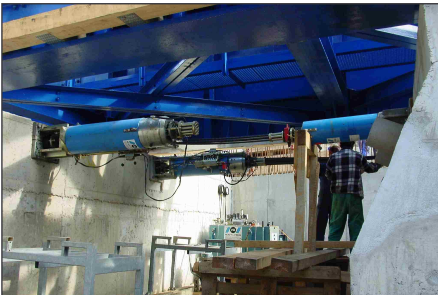
▲ VSL launching equipment installation, synchronized pulling and retaining strand jacks.
