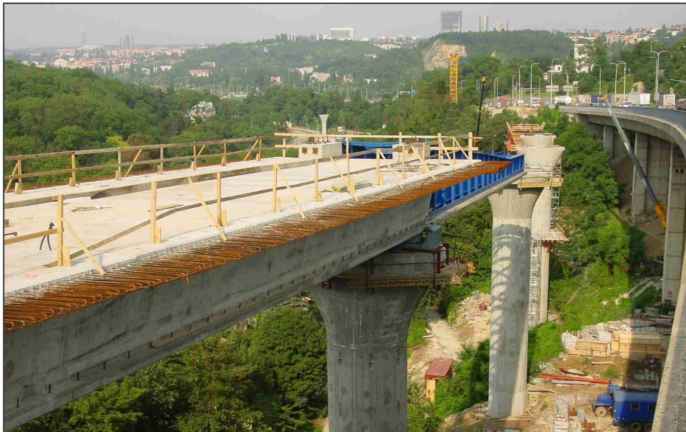
▲ View in bridge launching direction.
