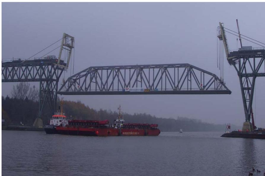
Formerly the Hochdonn railway bridge was the one that put limits to the height of the ships. Among the special features of the new construction is an increased clear height of 42m underneath the main span, to be par with the other bridges over the Kiel Canal. To achieve this increase of half a meter, the rails had to be installed directly on the steel structure.
