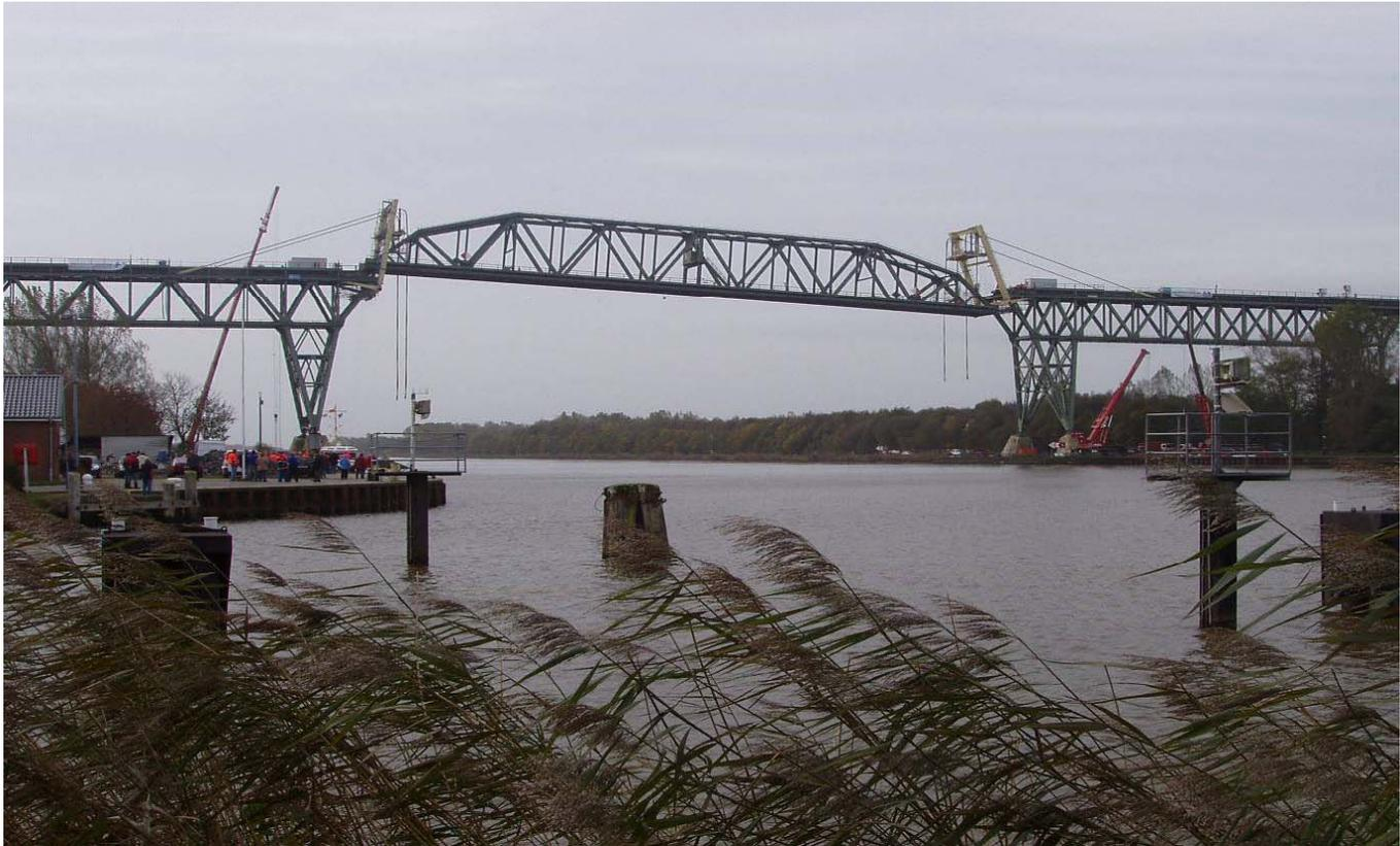
▲ *Shifting old part of the bridge to pass through existing supports*
