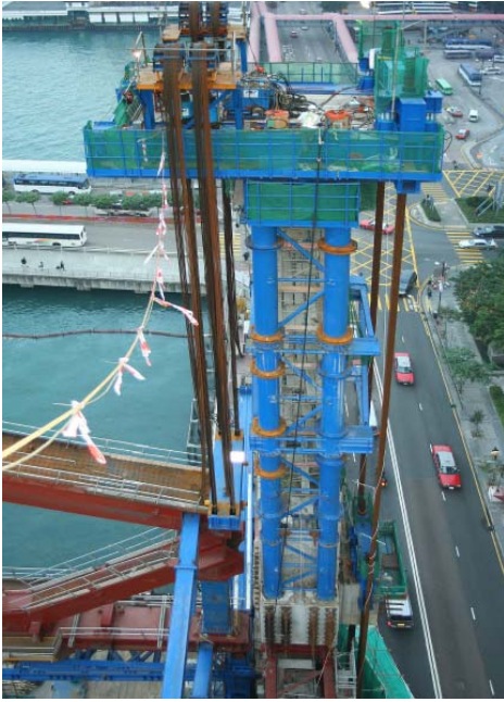
The self-balancing lifting bracket on column D/24
