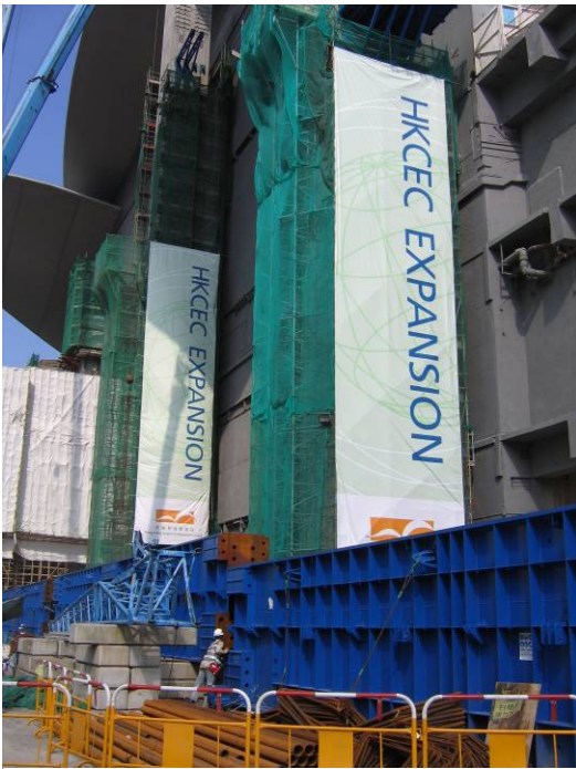
Hong Kong Convention and Exhibition Centre Expansion Project
