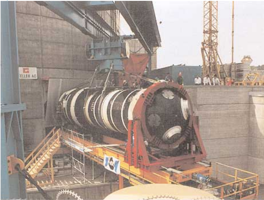
▼ SG being placed onto sliding carriages outside of the containment.
