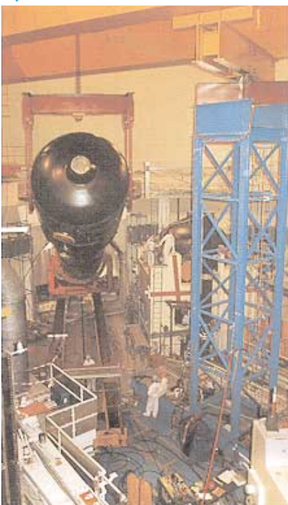
▼ Temporary support for polar crane.
