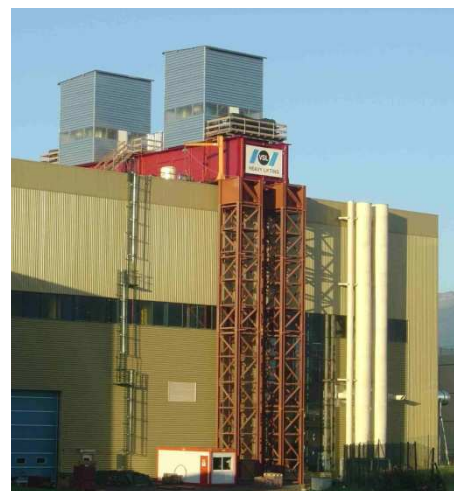
▲ Gantry with weather protections
