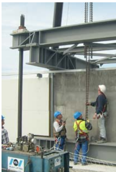
▲ Suspension of the roof during lifting
